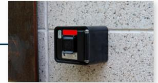
Rapid access key boxes eliminate the need for forced entry, minimizing critical delays, injuries and property damage
