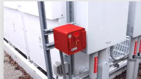
Remotely operate a shunt trip breaker to safely remove or isolate power from a building or equipment
