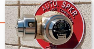
Locked FDC caps protect against damage, vandalism and debris
